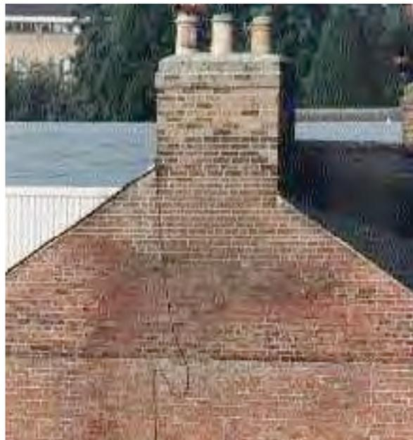
Condensing gases within a flue and terminal can have a corrosive effect on certain materials.
